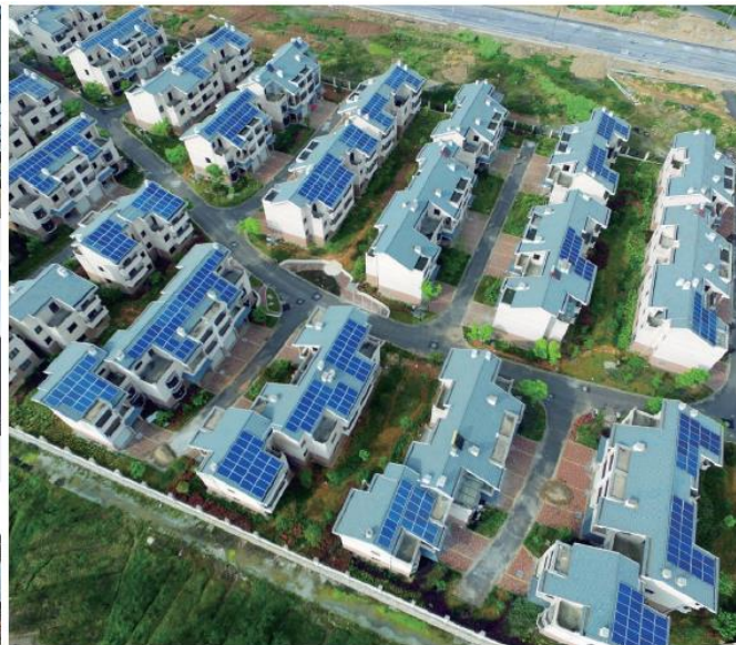
Quzhou Wecheng District 63 Residential Solar Systems 343kW
